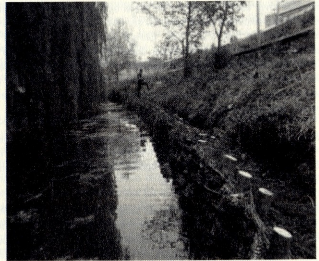
Figure 4: Installing stakes to protect the river bank form erosion.
