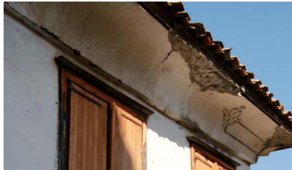
Figure 17: Eaves Covered with Wood Lath (a) or Lime Plaster (b) (Photographs by author, 2012)
