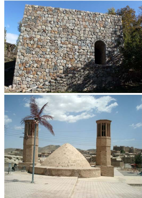
Figure 10: The simple structure of the crypt of Kordasht in cold and dry area (Top) as opposed to the complicated water reservoir with wind catchers in Naeen (Bottom) in the central arid zone of Iran
