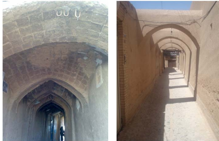
Figure 9: Sabat or roofed passage in Kashan (Left) and a narrow passage with bracing arches in Yazd which provide sheltered pathway for the pedestrians
