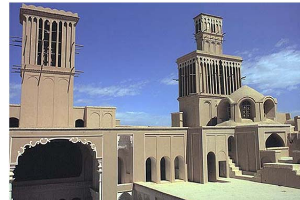
Figure 13: Use of domes and self-shading forms in Agha Zadeh House in Abarkuh, Yazd
