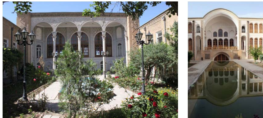
Figure 3: Qadaki house in Tabriz (Left) with small central courtyard and flat roofs as opposed to Aameriha house in Kashan with very large central courtyard and arches and domes
